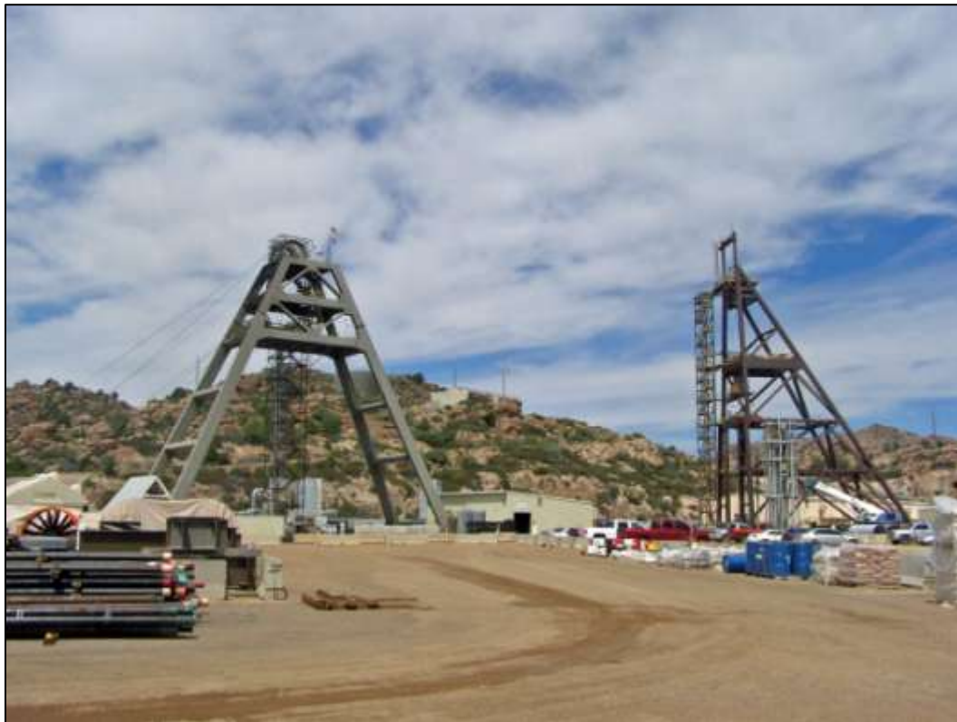
No. 10 (left) and No. 9 Shaft (right) at the East Plant Site looking west (June 2015)
