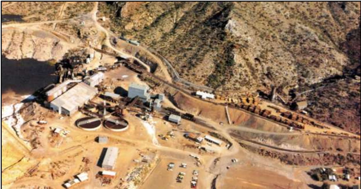
Aerial View of the Magma Copper Concentrator (Photo by Magma Copper Company)
