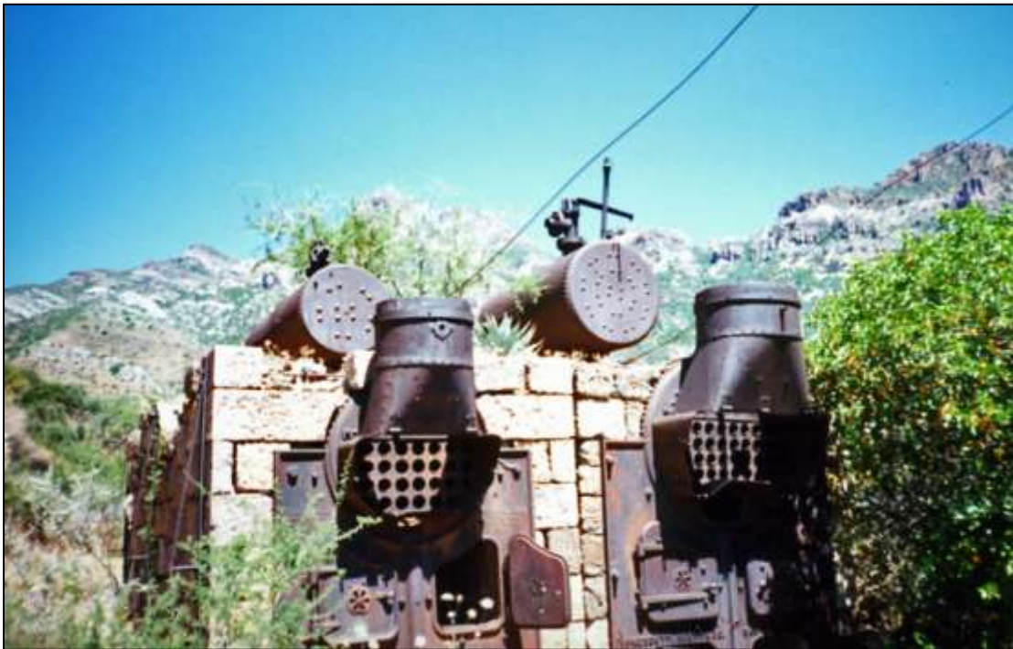
Old Boiler at Silver King Mine Site near Superior, Arizona
