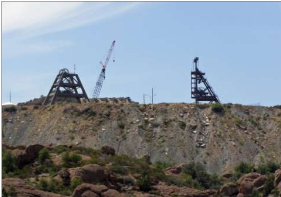
Resolution Copper's 6,943-foot No. 10 Shaft (left) is the Deepest Single Lift Shaft in the United States (Photo by David F. Briggs, August 2009)
