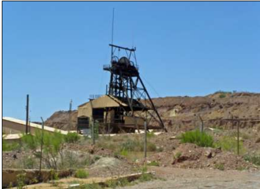
Junction Shaft is located along southeast rim of Lavender Pit.
