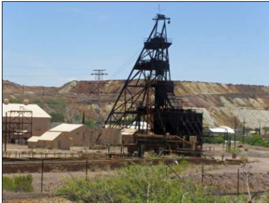
The Campbell Shaft is located about 0.5 miles southeast of Lavender Pit.
