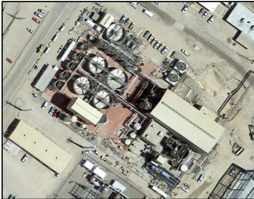
Concentrate Leaching Facility at Morenci, Arizona (from Google Earth - 5/9/2014)
