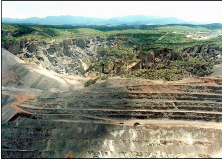
Open Pit at San Manuel, Looking South toward Santa Catalina Mountains on Skyline. Broken Ground in the Far Wall Resulted from the Collapse of Surface Exposures above the Underground Block Caving Operation (Photo by David Briggs, early 1990s).
